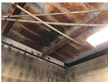
Pool Pump Room
