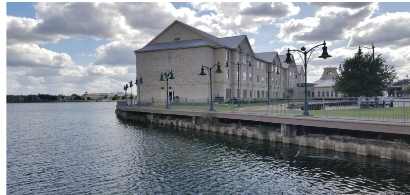
Granbury Convention Center and boardwalk on Lake Granbury.
