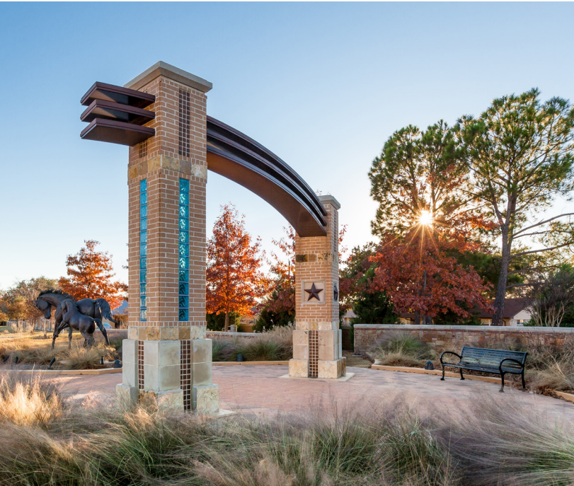
MacArthur Gateway Arches in Irving.
